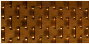
3. Illuminated timber lining Warm timber with concealed LED
